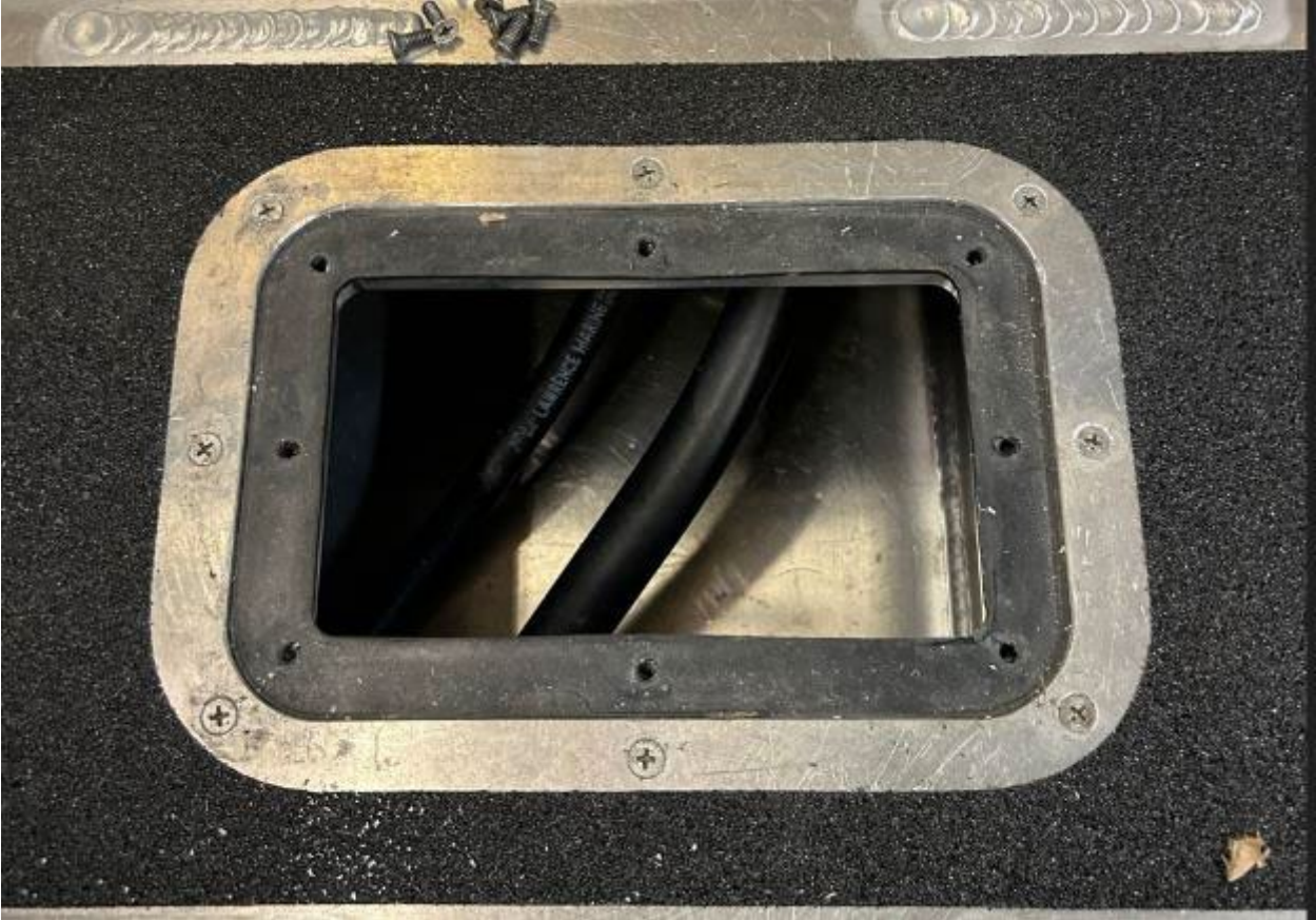
Figure 5: Hatch opening with access lid removed.
